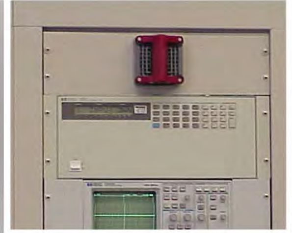
Close-Up of Safety Lamp that Flashes when HIPOT is in use
